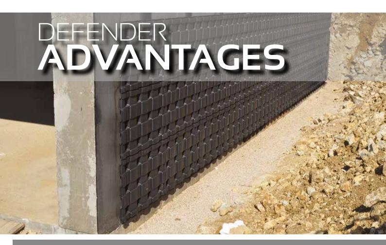
It combines the advantages of dimpled membrane and gravel, suitable for better protection of the waterproofing and ventilation of the basement walls
